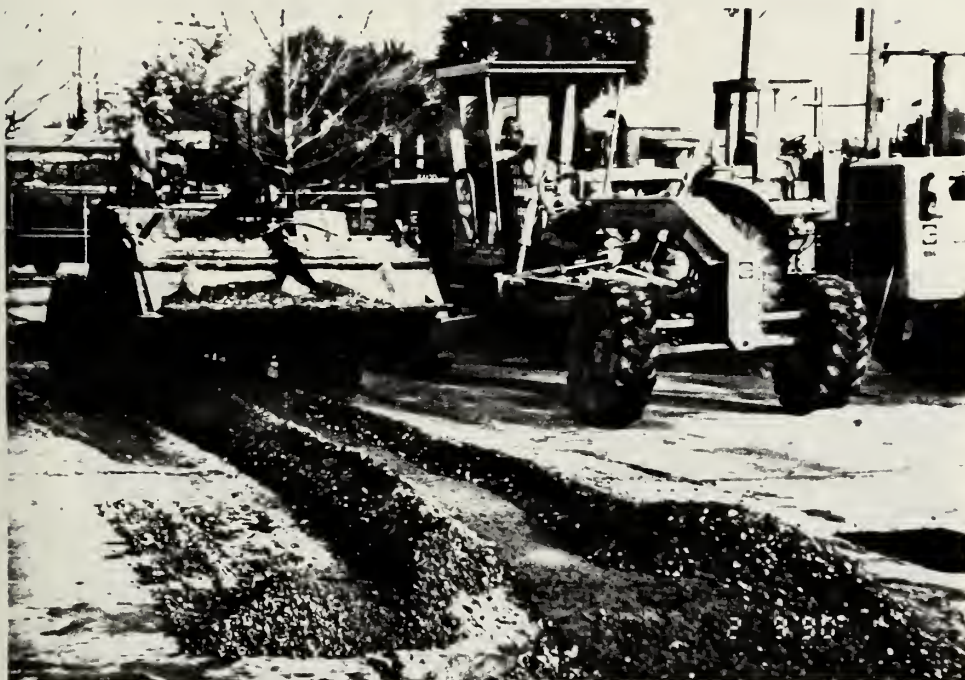
Figure 2.17 Repositioning Soil Stabilizer
